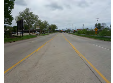
Much of Chicago Drive in the study area consists of five vehicular travel lanes.
