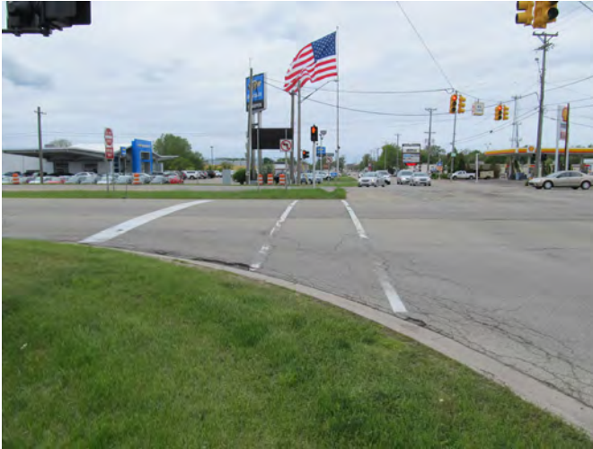
US-31/8th Street intersection before potential improvements.
