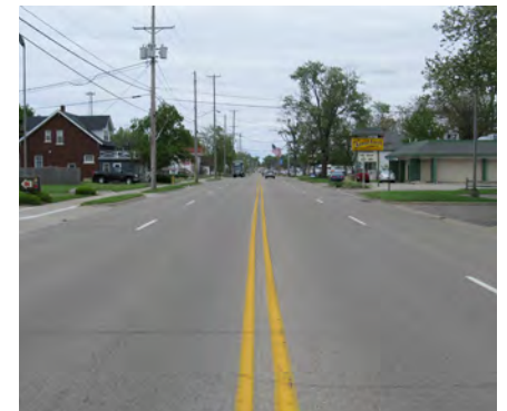
8th Street in the study area consists of four vehicular travel lanes.
