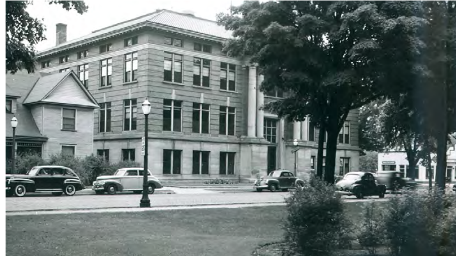
Historic photo of Holland City Hall, from the City of Holland.
