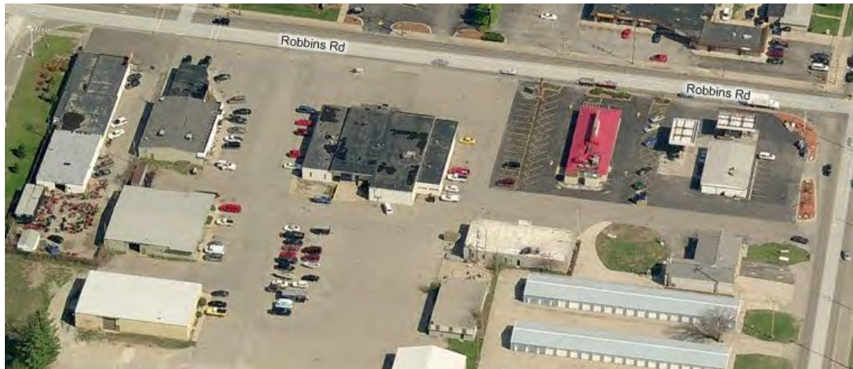
The lack of definition within the parking areas may lead to confusion for drivers and an unsafe environment for pedestrians
