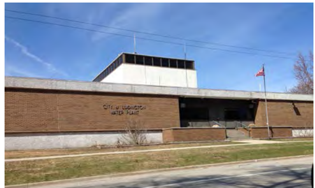
Ludington's water treatment plant, located on Lakeshore Drive.
