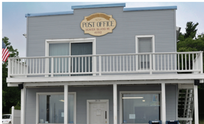
The United States Postal Service operates daily mail service through the Beaver Island Post Office and Island Airways. The Post Office building is a unique and historic structure located in downtown St. James.
