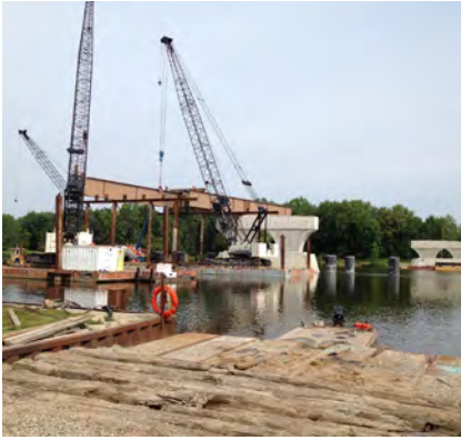
US 31 Bypass, under construction
