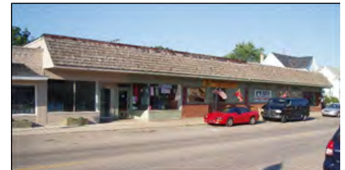
An example of an applied mansard roof frequently used to update older commercial buildings in the mid 20th century.
