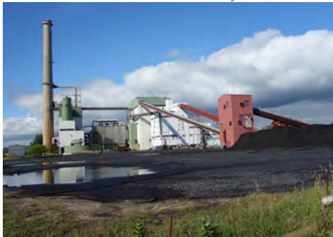
The Sims Generating Station Unit III consumes 550 tons of coal each day
