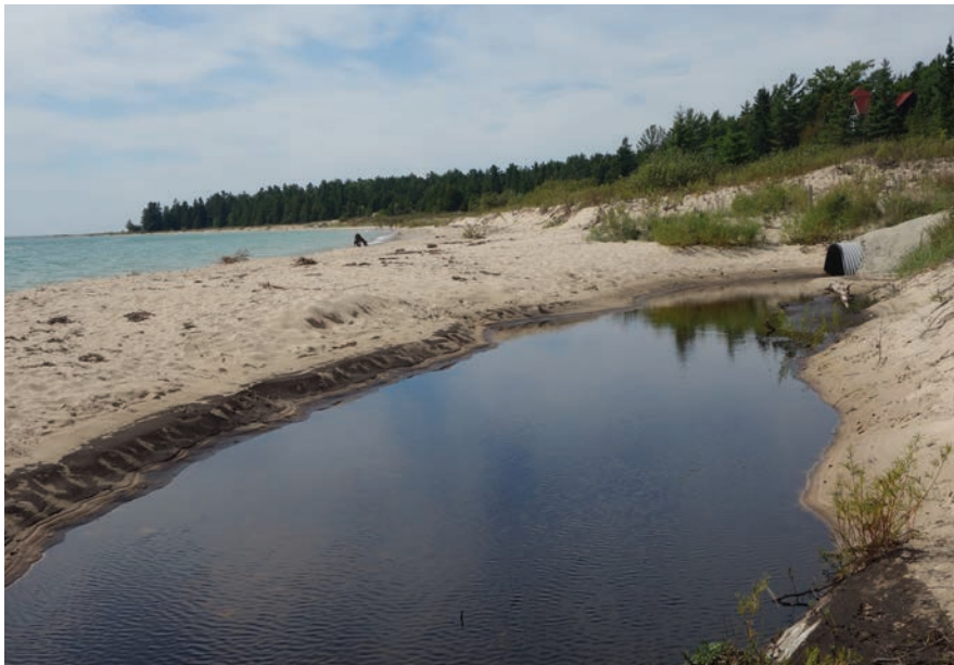
The Charlevoix County Road Commission also maintains the culverts and infrastructure that supports the Island's roads.
