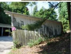
This condemned structure in Grand Haven Charter Township has been damaged by the natural movement of dune systems over time. Homes within the shorelands may be subject to erosion, sand movement, and other coastal dynamics.
