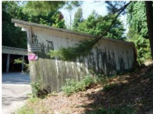
This condemned structure in Grand Haven Charter Township has been damaged by the natural movement of dune systems over time. Homes within the shorelands may be subject to erosion, sand movement, and other coastal dynamics.
